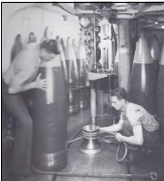
**Seaman A. Longley & Gunners Mate 1st Class H. Castles use a power-driven rotating capstan & a piece of line to parbuckle a projectile in turret two barbette (9 April 1953)**
