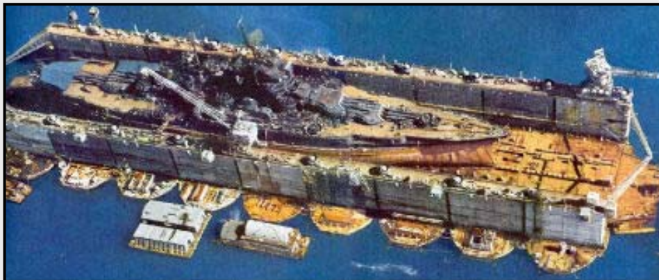
(Official US Navy Photo. USS IDAHO (BB-42) in ABSD (Advanced Base Sectional Dock))
