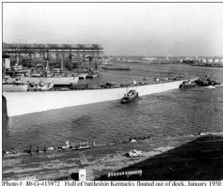
Photo # 80-G-413972 Hull of battleship Kentucky floated out of dock, January 1950
