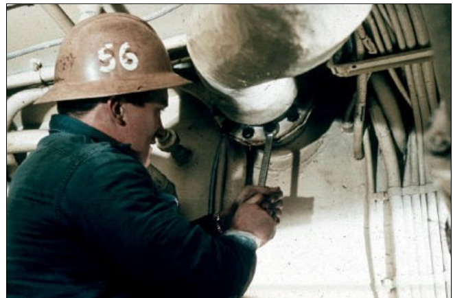
Shop 56 - Pipefitters and Wrappers
