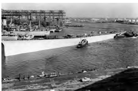
U.S. Navy photo (USNHC #80-G-413972), shows the hull of BB-66 being floated out of dry dock on January 20, 1950
