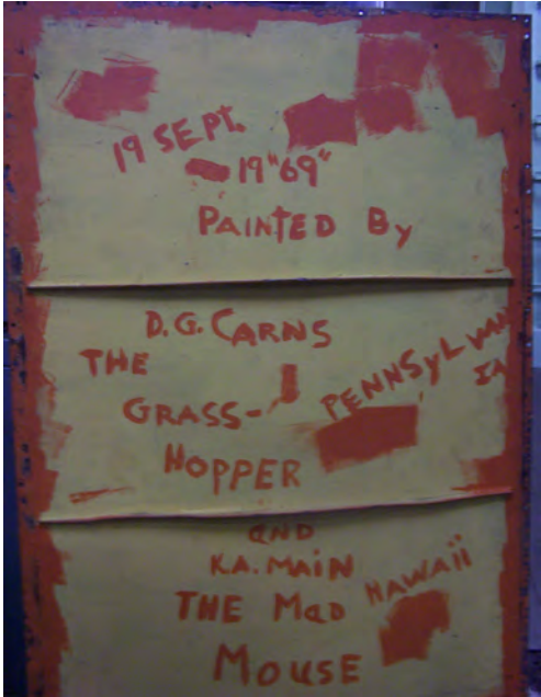
Messages painted on underside of deck plates in Forward Plot
