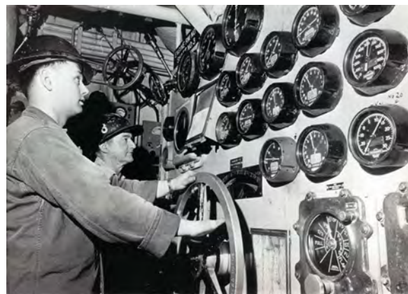
Civilian engineers watch gauges as they start main engine #3 on February 24, 1968. This was the first time the engine had been started in over ten years. AP Wire photo, courtesy of Ron Reeves, HTC, (ret.)
